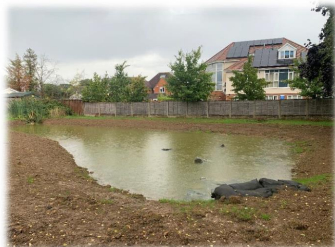
(below) a holding pond to store excess water at a low part of the park
