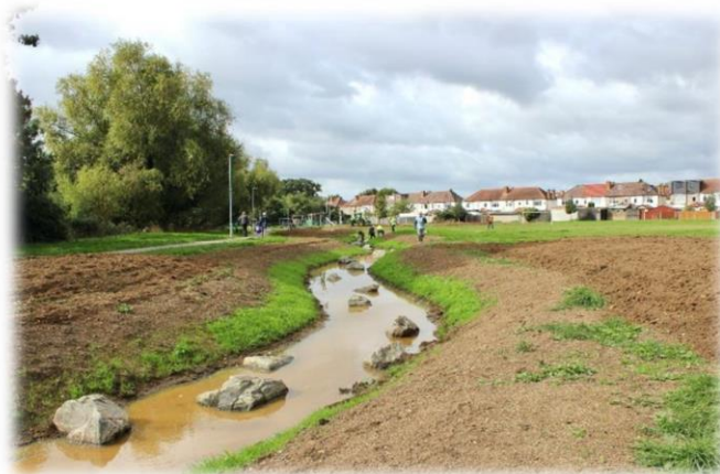
(above) A swale on a naturalised path that will become a significant biodiverse feature when planting matures
